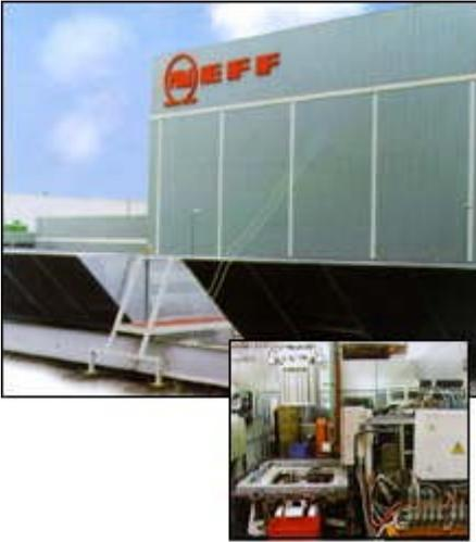
Waste air from compressor cooling is carried away by weatherproof ducting.
