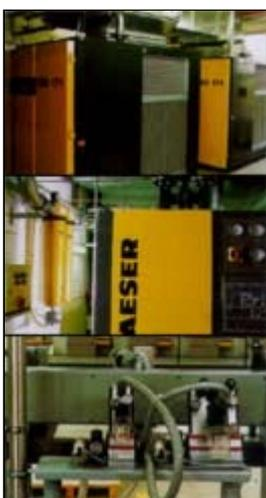
The compressed air center equipped with four KAESER screw compressors, booster and air treatment plant (upper and center).
