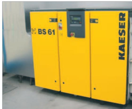
the brewery operates a total of 17 energy efficient KAESER screw compressors all controlled by KAESER's PC-based compressed air management systems. Air treatment and filtration precisely tailored to meet the brewery's requirements guarantee the constant and critical air quality required by the brewing process.
