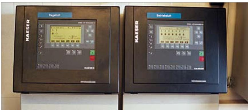
**Both of the compressed air systems, which are housed in facilities also supplied by Kaeser, are controlled via two "Sigma Air Managers"**
