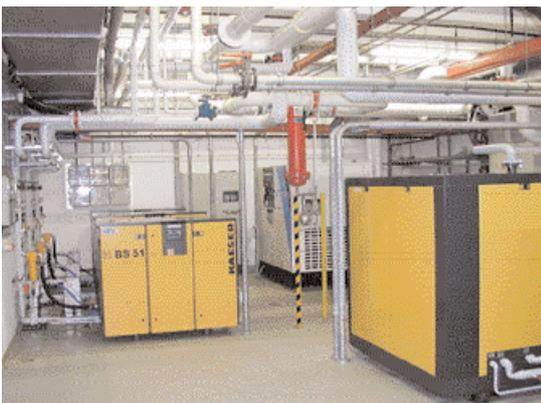
is a variable speed drive machine and functions as a peak load compressor. The advantage of the SFC system is to be found in its fine matching to the actual air demand. A VESIS controller that ensures even loading and efficient operation of the compressors was also included. To further improve energy balance, the BS machine was supplied with a heat recovery system providing hot water, for which there is an annual requirement of 600 cubic metres.
