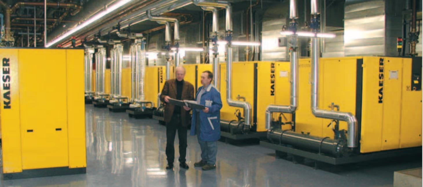
**The new centralised compressed air system**
