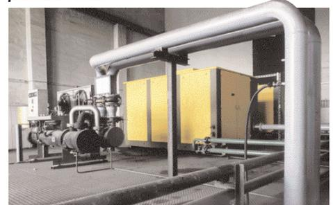
*The 10 kV power supply is transformed down to 5 kV for the compressors*
