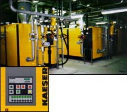
In the air center, seven KAESER screw compressors with state-of-the-art air treatment and control engineering are installed.
