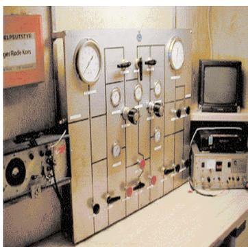
***Underwater operations are monitored and controlled from the control room while the compressor room houses the complete air generating and treatment plant***
